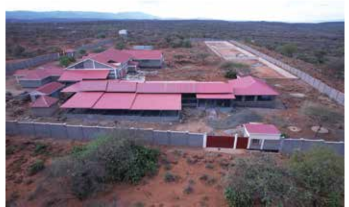
Shs. 200 million Export Abattoir at Maoi in Baringo South (90% Complete)
