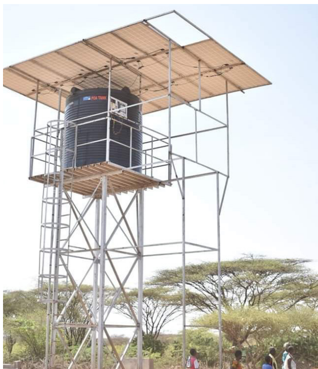
An overhead water storage and distribution tank in one of the solar-powered borehole projects.
